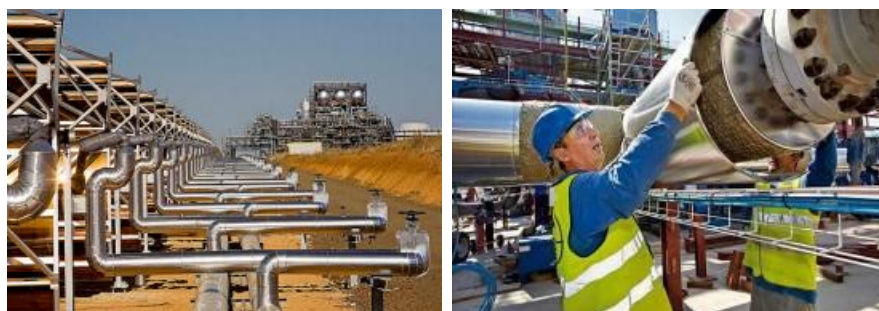
Figure 71 Solar field piping; one header pipe transports the cold oil to collector, the second header pipe transports the heated oil back to the power block; (source: Estela Solar, 2010); Assembly of the piping (BilfingerBerger, 2010)
