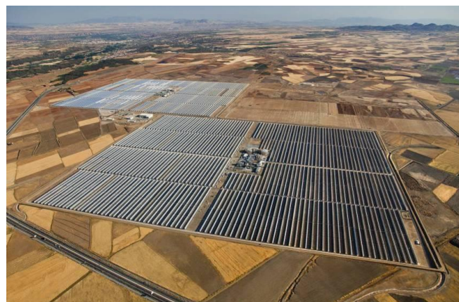
Figure 4 Parabolic trough power plants Andasol 1 (front) and Andasol 2 (rear) in Spain with a capacity of 50 MW each and a storage size of 7.5 full-load hours. The power block and the storage are in the center of each solar field.
